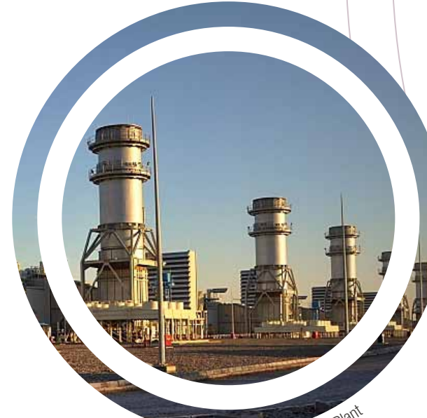
Nainawa Power Plant
